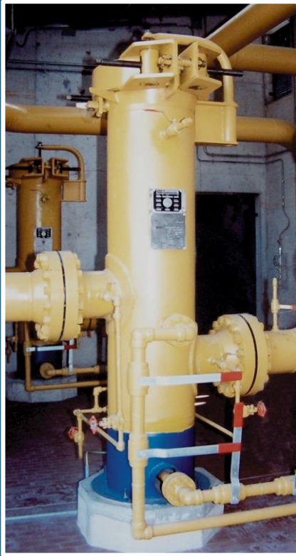
2 GAS FILTERS FCV TYPE - 20" # 600
