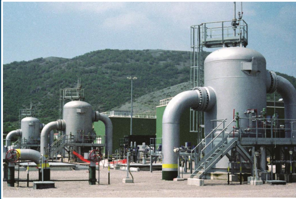
3 SC TYPE MULTITUBE SEPARATORS - 130" # 600 THK. 90 mm, 90 Ton each
