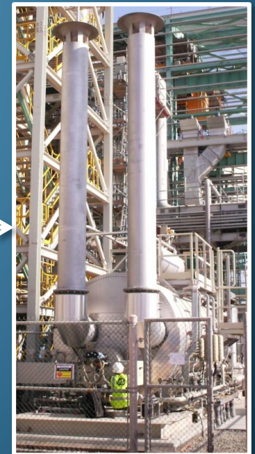
FORCED DRAFT OIL BATH HEATER 4.500.000 KCAL/h
