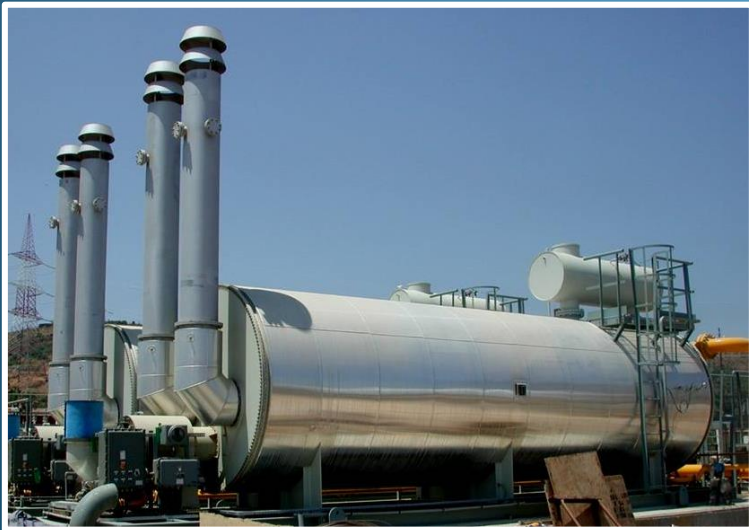
2 FORCED DRAFT WATER BATH HEATERS – 3.900.000 KCAL/h each
