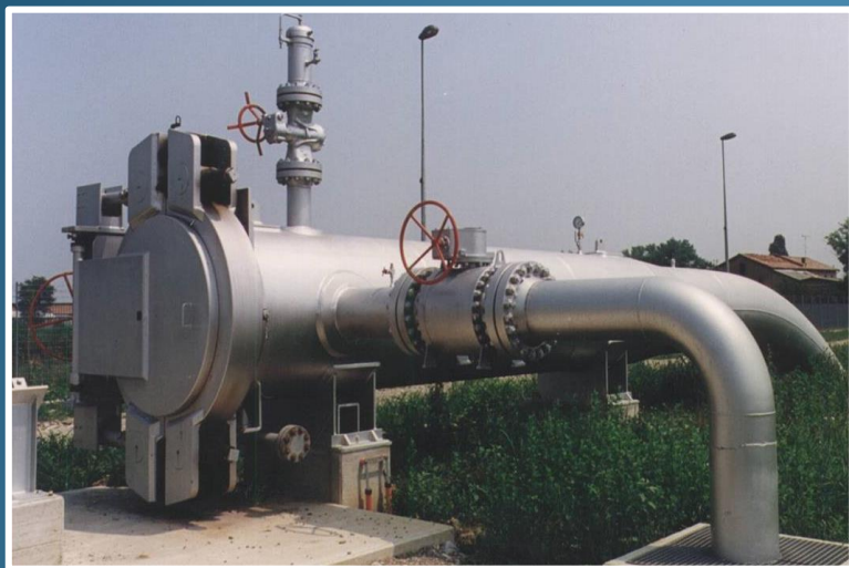
BIDIRECTIONAL TRAP 48" x 56" # 600
