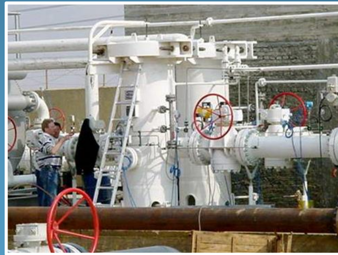
2 GAS FILTERS FCV TYPE - 34" # 600
