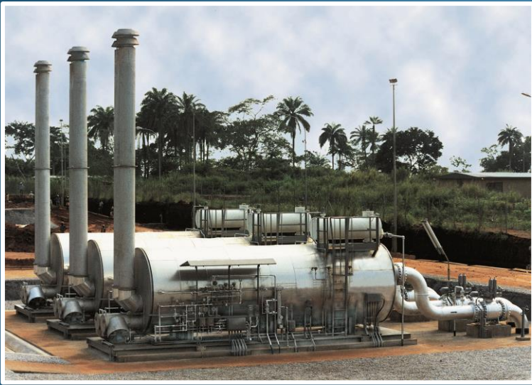
3 NATURAL DRAFT WATER BATH HEATERS – 2.000.000 KCAL/h each
