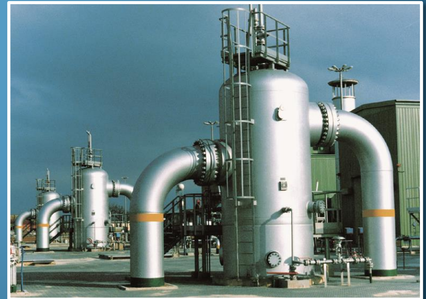
3 SC TYPE MULTITUBE SEPARATORS - 96" # 600 THK. 75 mm, 45 Ton each
